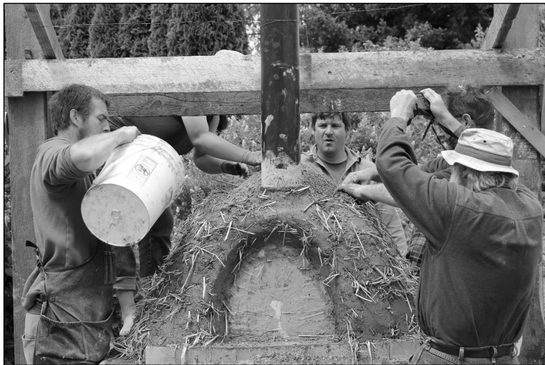
Cob-oven building workshop using materials from the farm
